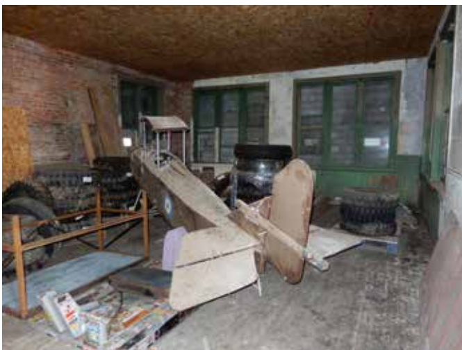
View of classroom showing original windows.
