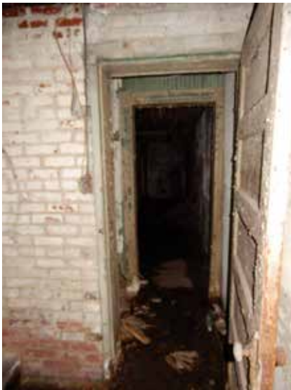
View of basement.
