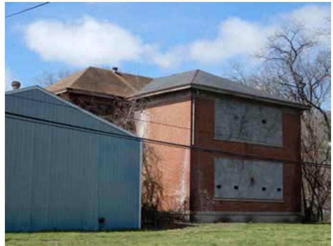
View of rear addition with slate roof and blocked up windows.
